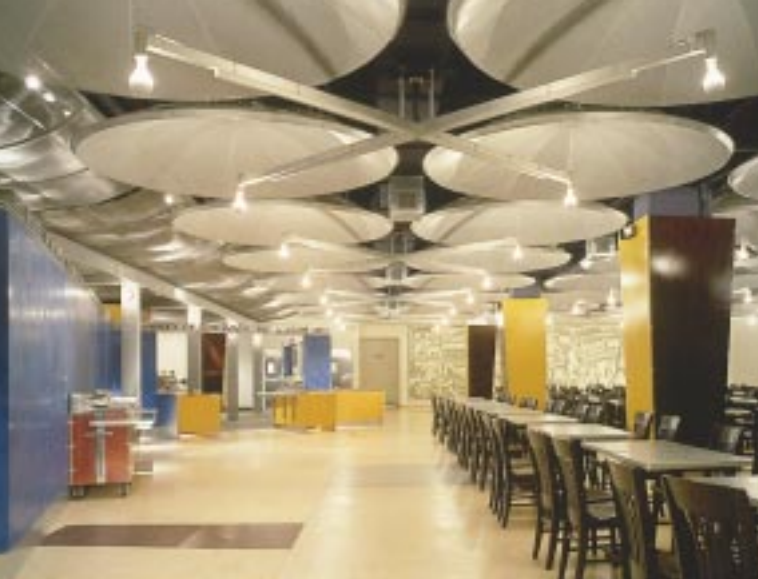
The Market at Newport is an office food court with the feel of an open-air market. (left, top & bottom) The solution was to develop large-scale “umbrella” luminaires that double as the ceiling system. A silver-bowl lamp originating at the focal point of a parabolic contour re-directs light for a more efficient use. The silver bowls also control glare.
